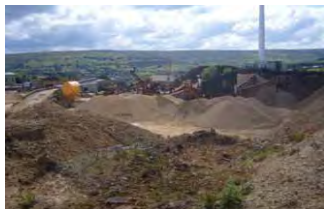
Screening Plant, Naylor Hill quarry
