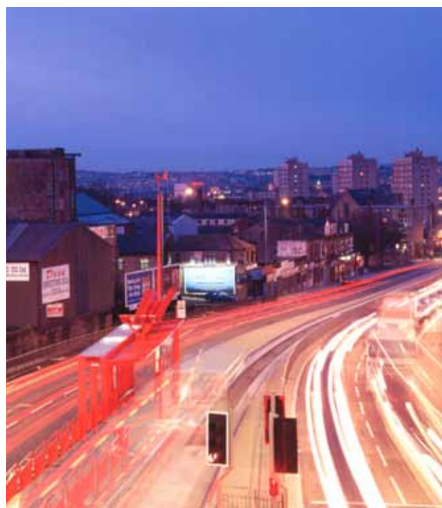
Guided bus lanes, Manchester Road, Bradford city centre
